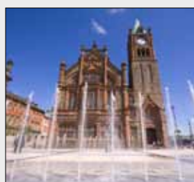
FP McCann | DSD's Derry City Public Realm Project, Northern Ireland
